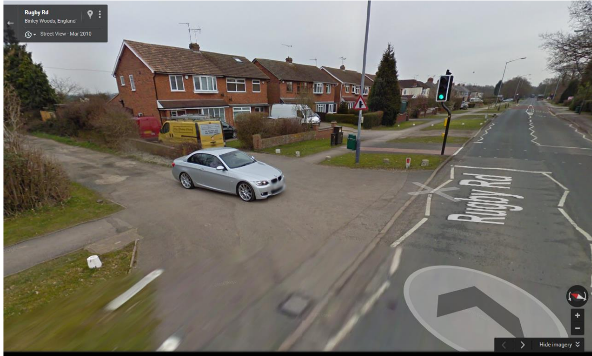
Photo1 – Looking east along A428, access road on left from A428 leading to site boundary
